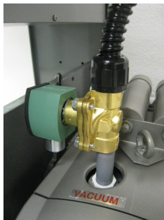
Air Valve Assembly
